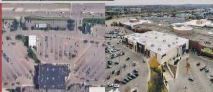
PACIFICA BURNSVILLE (RENOVATION & NEW CONSTRUCTION)
