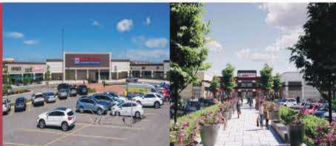
PACIFICA SQUARE (RENOVATION & NEW CONSTRUCTION)
